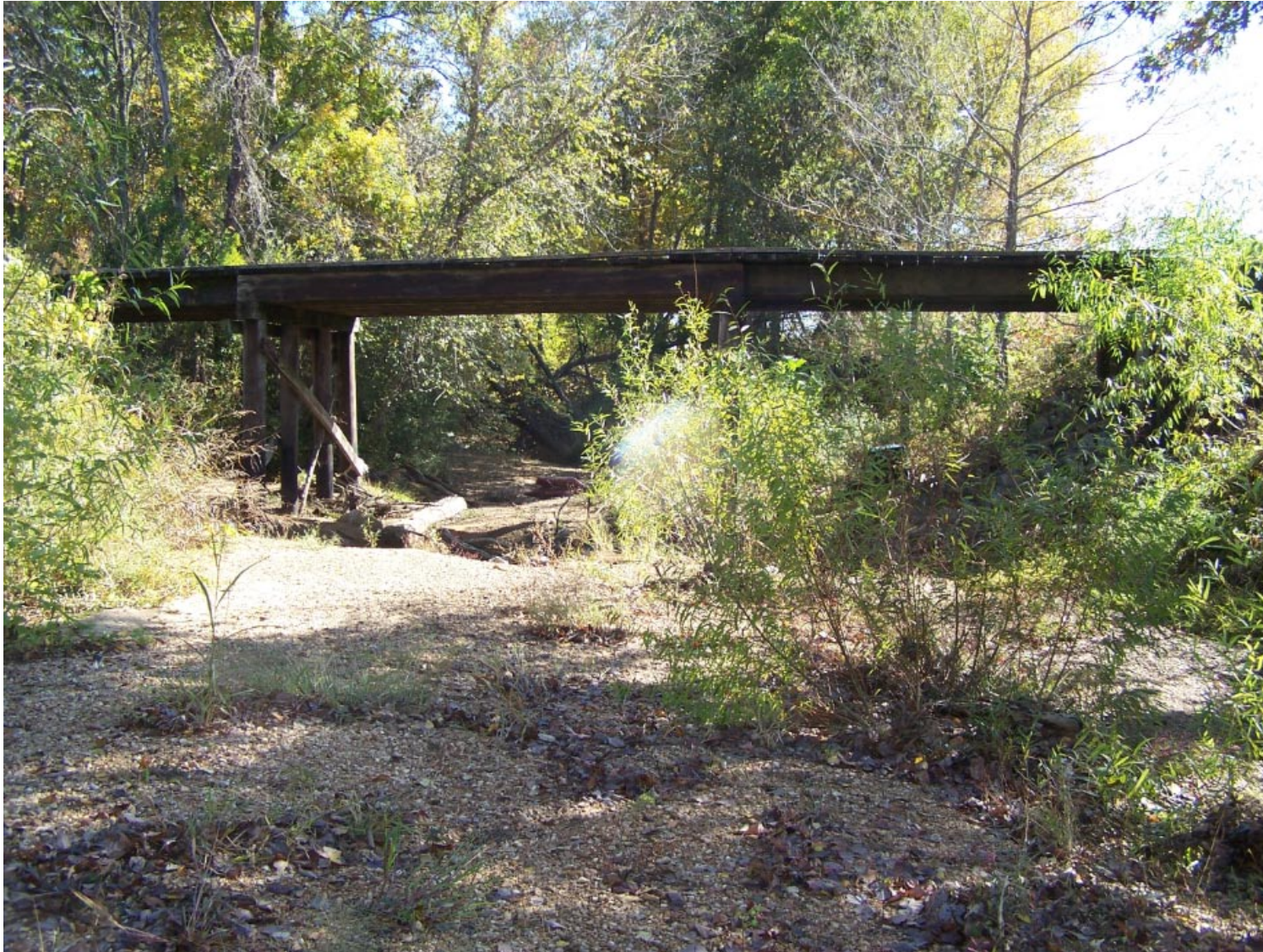
042-C252 UPSTREAM SIDE 10/20/2011
