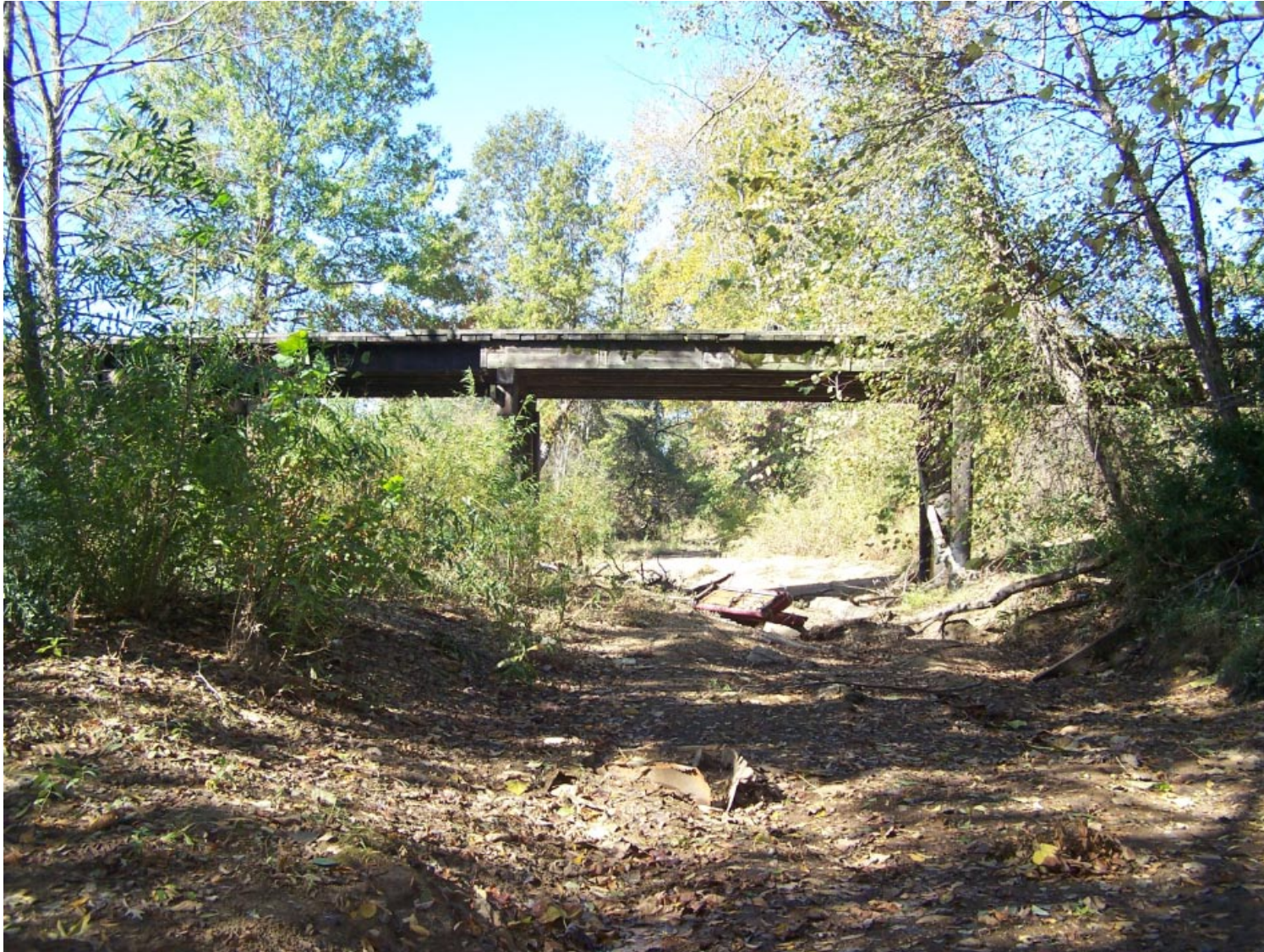
042-C252 DOWNSTREAM SIDE 10/20/2011
