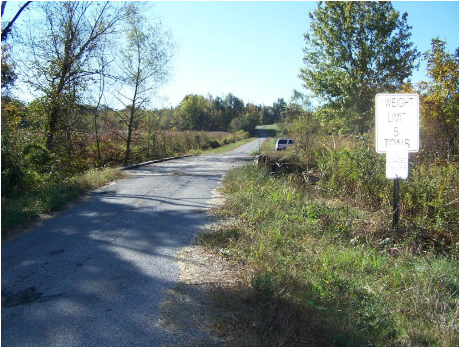
042-C252 LOOKING SOUTH 10/20/2011
